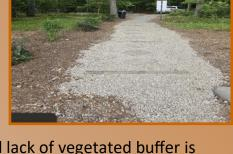
**Problem**: Stormwater runoff and lack of vegetated buffer is causing minor erosion at the Shapleigh Town Beach, causing pollutants to enter adjacent Square Pond. Foot traffic compacts the soil and runoff cannot infiltrate so is exacerbating erosion issues.
